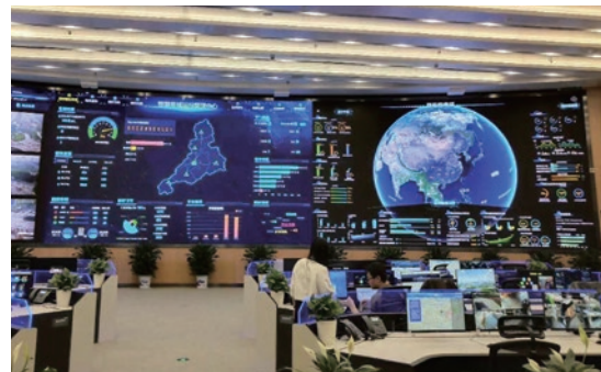
Smart City Control Center In Jinan, China
