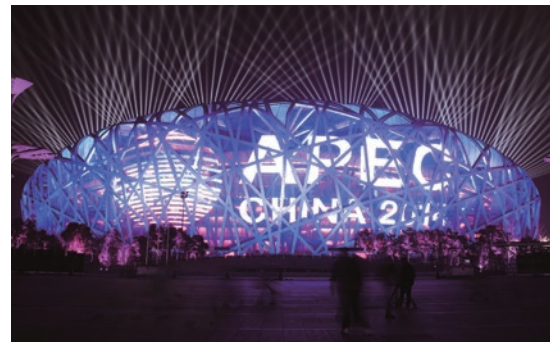
National Stadium Bird's Nest, China
